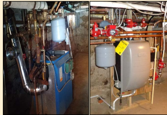
Before & After Boiler Replacement
